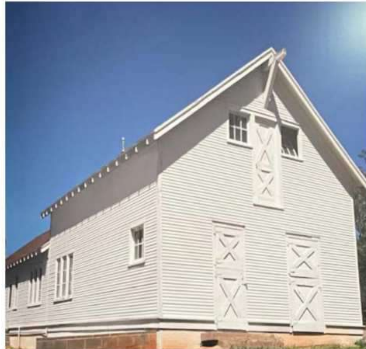
Ranger Station Barn
