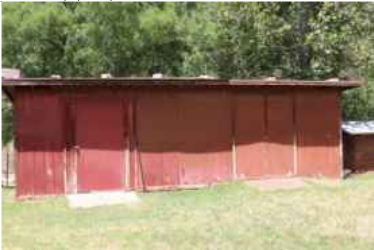
Equipment Shed, 115 Schnebly Hill Road
