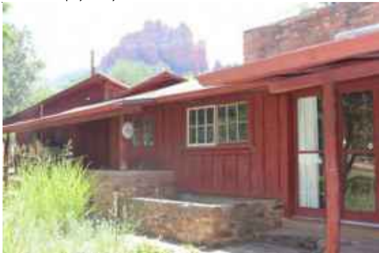
Dwelling, Rear Elevation, 95 Schnebly Hill Road
