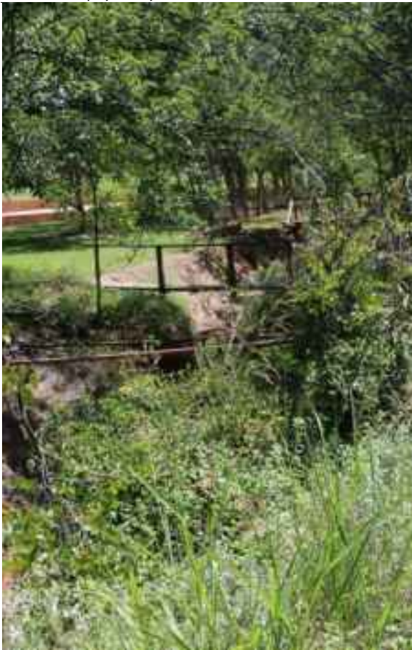
Dry Wash and Piping for Farley/Steele Ditch, 95 Schnebly Hill Road
