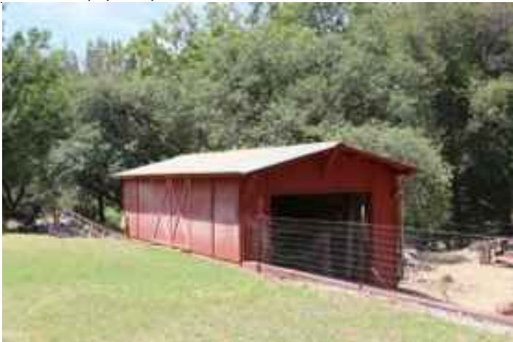
Storage Barn, 115 Schnebly Hill Road
