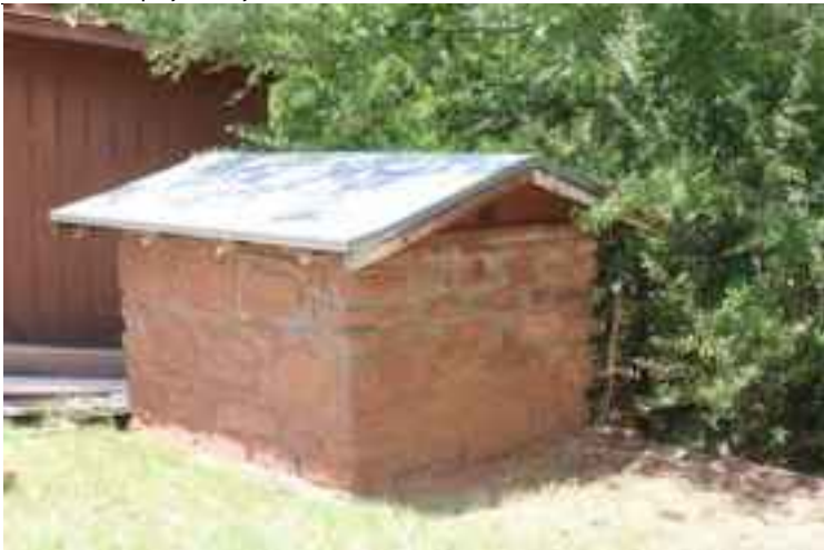
Historic Water Storage Tank Building, not in use, 115 Schnebly Hill Road
