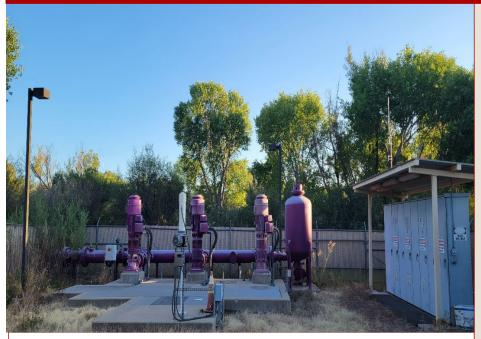
The existing recharge well filter system utilizes disposable filters, resulting in excess cost and waste for filtration. This project will replace the existing filtration system for the recharge well pump station with a new backwash filtration system.
