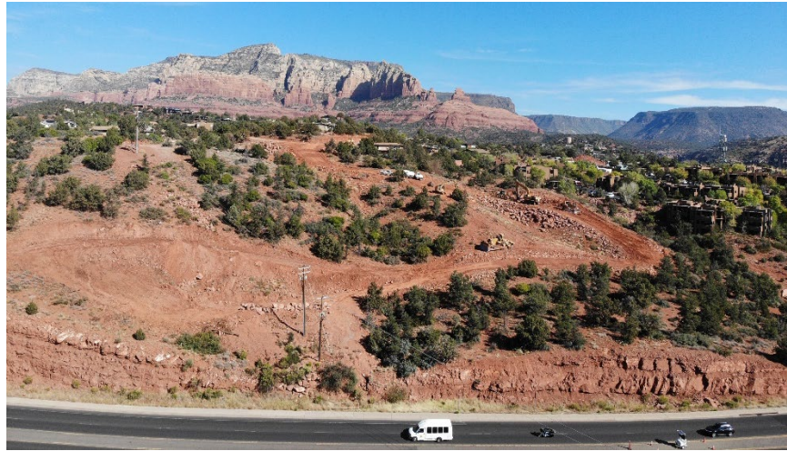
Recent View of Forest Road Extension Project
