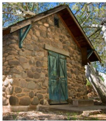
7. Hart Pump House
