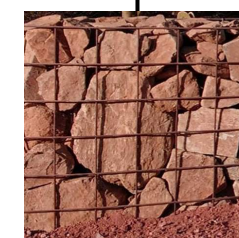
Rock Gabion Walls
