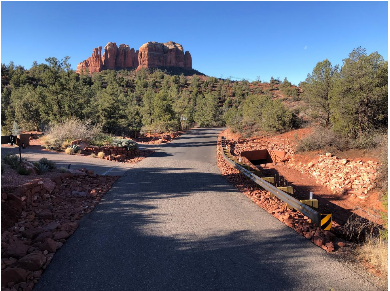
Back O'Beyond Crossing – Project completed August 2023
