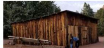
Jordan Ranch Tractor Shed
