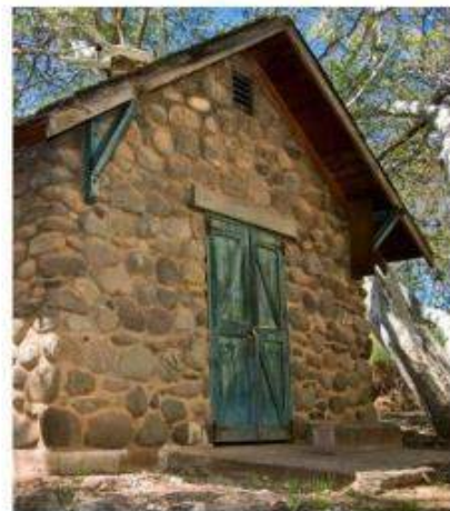
7. Hart Pump House
