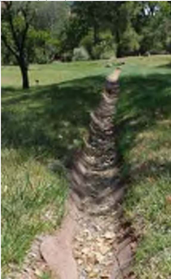
Cement Lined Section of the Farley/Steele Ditch, 105 Schnebly Hill Road
