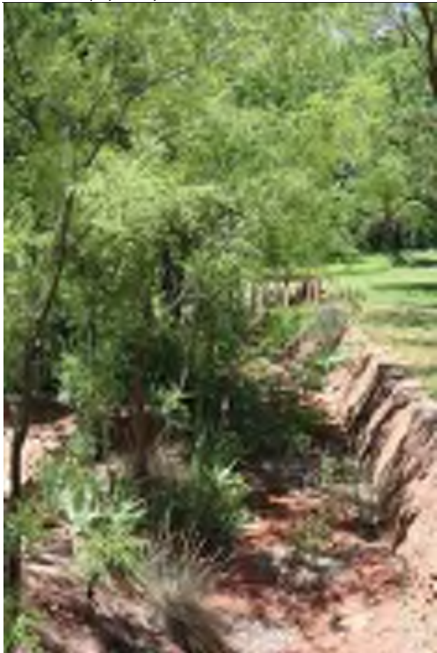
Rock Lined Section of Farley/Steele Ditch, 105 Schnebly Hill Road
