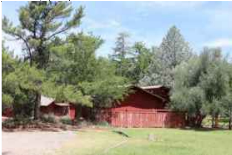
Converted Garage and Main Dwelling, 95 Schnebly Hill Road
