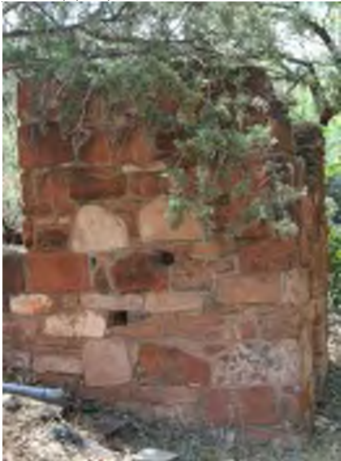
Seep Well Housing, 65 Schnebly Hill Road
