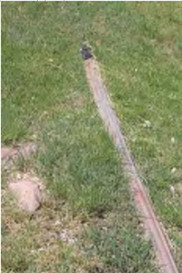
Corrugated Pipe Section of the Farley/Steele Ditch, 105 Schnebly Hill Road
