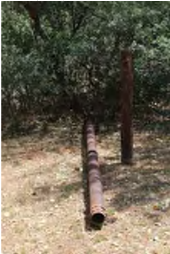
Support Post and Section of Raised Pipe, 105 Schnebly Hill Road
