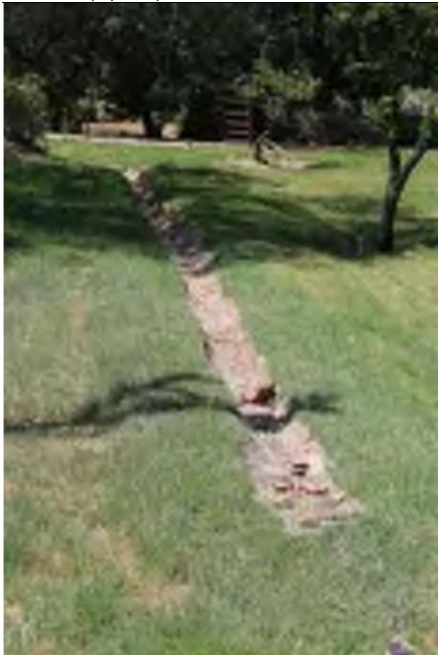
Concrete Lined Section of the Farley/Steele Ditch, 105 Schnebly Hill Road
