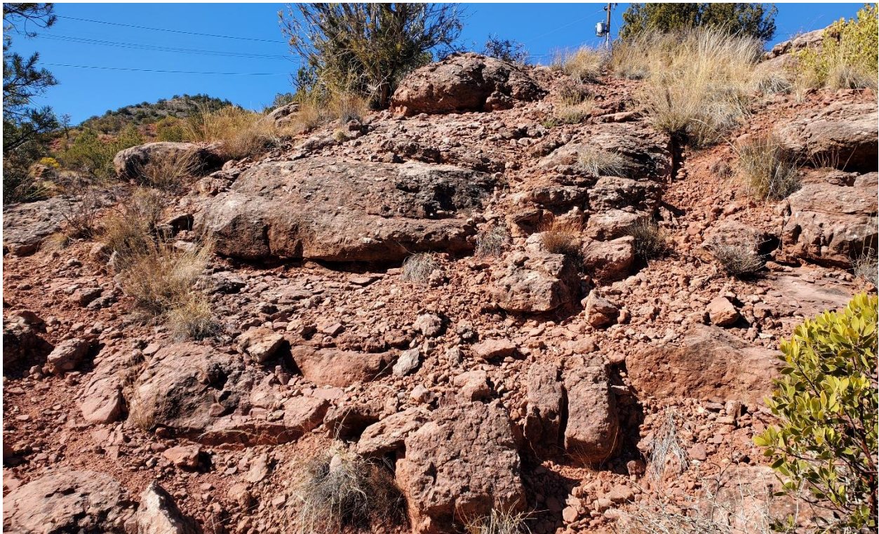
Figure 4: General site conditions showing ledgy rock outcrops and over-sized aggregate (particles greater than 3.0 inches)
