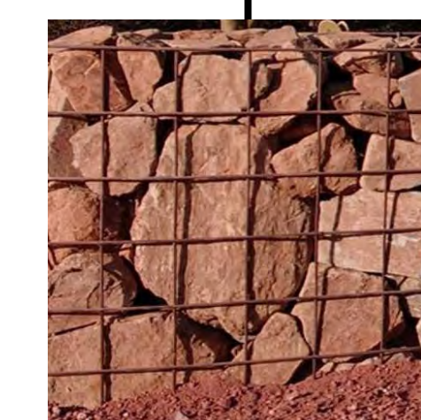
Rock Gabion Walls
