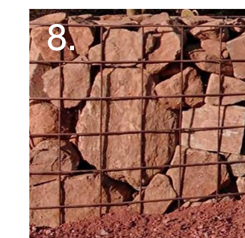
Red Rock Gabion Walls
