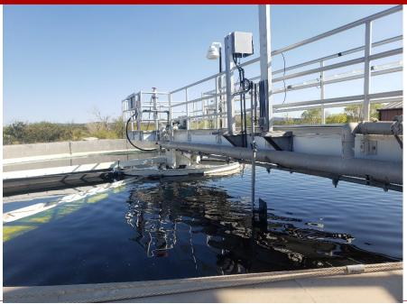
This project will replace the existing original clarifier mechanisms with new mechanisms consisting of a new drive system, skimmer arm, counterbalancing arm, suction header, and weir washer. It will also repair any damage to the clarifier coating that as occurred from off-balance mechanisms.
