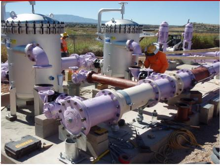
The existing recharge well filter system utilizes disposable filters, resulting in excess cost and waste for filtration. This project will replace the existing filtration system for the recharge well pump station with a new backwash filtration system.
