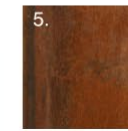
5. Sweeping Metal Facade Corten Steel
