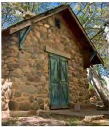
7. Hart Pump House
