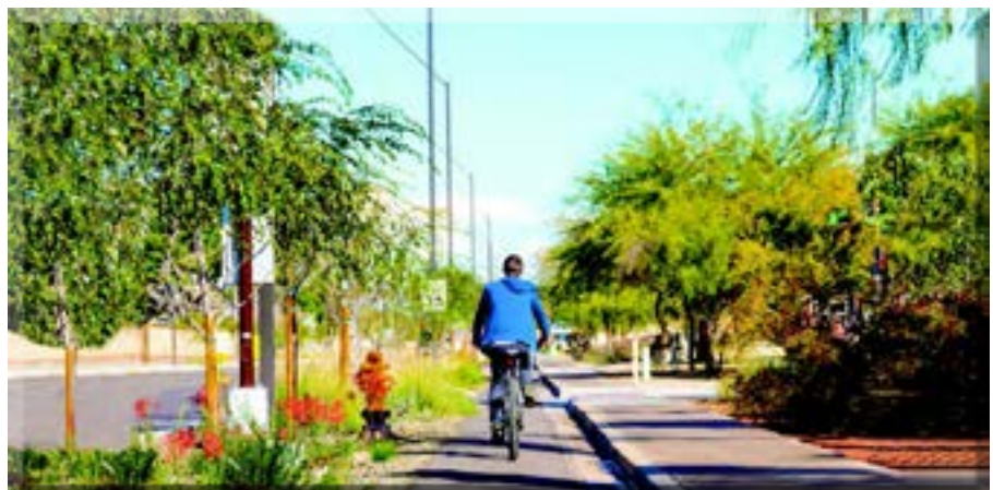
Figure 6.2. A Complete Street that features a “protected” bike lane with a landscaped buffer between the road, the bike lane, and sidewalk. Source: Avondale Community Sustainability Plan
