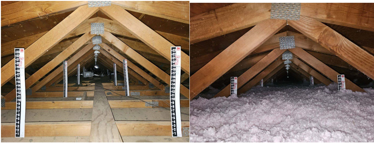
Figure 1: Before and After Insulation Repair performed by CozyHome
