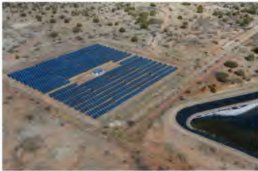
Wastewater Treatment Plant solar
