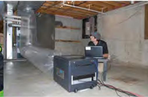
Building envelope/duct sealing
