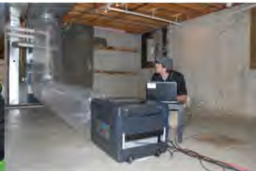
Building envelope/duct sealing
