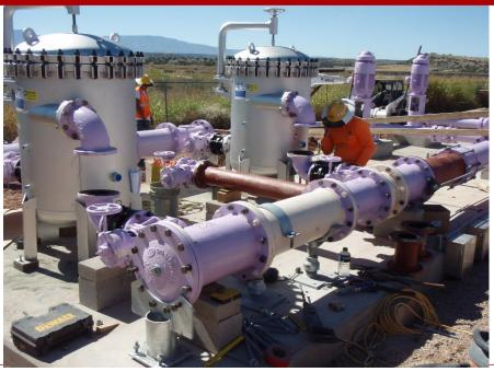
The existing recharge well filter system utilizes disposable filters, resulting in excess cost and waste for filtration. This project will replace the existing filtration system for the recharge well pump station with a new backwash filtration system.
