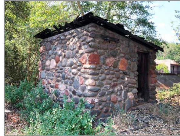
1939 George Jordan Wellhouse, 40 Art Barn Rd
