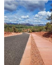
Hillside Vista Estates SUP
