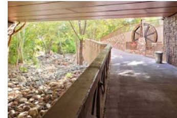
Pedestrian Undercrossing SUP at Oak Creek
